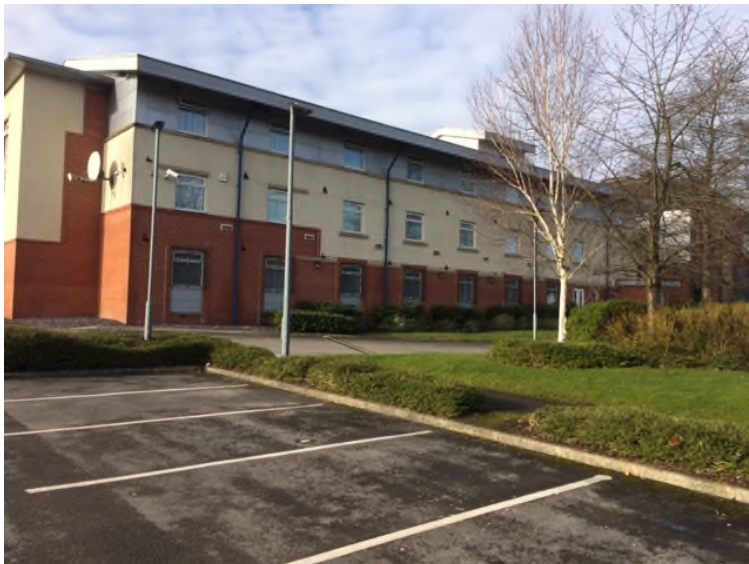
View of rear elevation of existing hotel and the area to be extended
